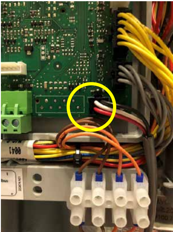
Cascade Cable Connection on INSTINCT Master Boiler
