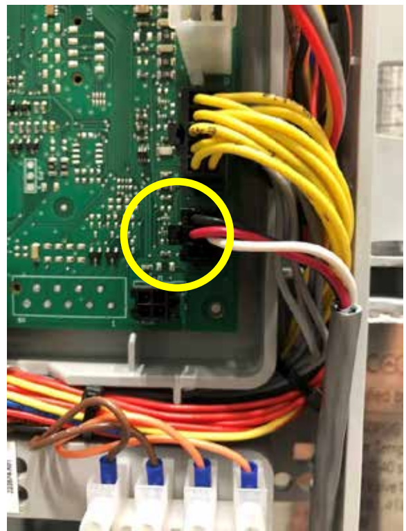
Cascade Cable Connection on INSTINCT Slave Boiler
